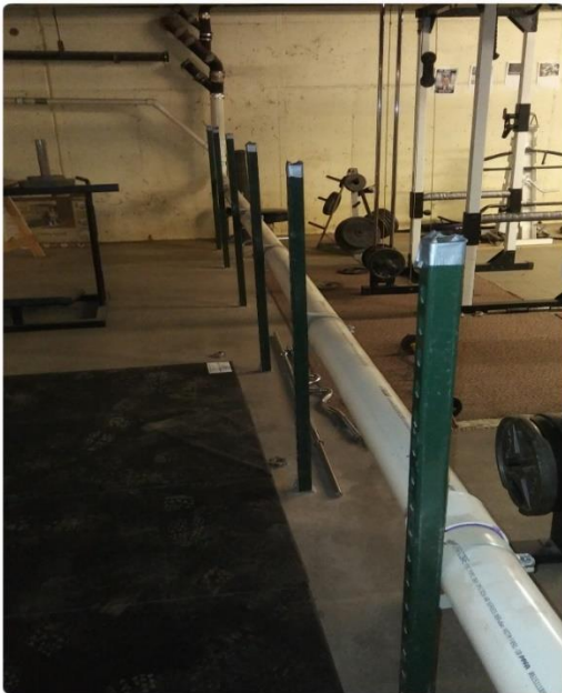
These photographs display the conditions of the plumbing in the jail area. Note that the cast iron has failed and has been replaced with PVC which is installed across the floor in the garage.
